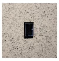
3. Insert the Smoothline wall flange. Glue the flange to the stone using a glue that is compatible with the solid surface. It may be easier to glue the flange in before installing the stone.
