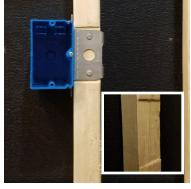
2. Complete the solid surface material installation, making sure the junction box is centered in the opening. The junction box needs to be at a depth that allows the wood system flange to end up flush with the solid surface.
